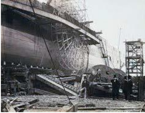
Figure 1 Chantier naval de John Scott Russell - 1858
